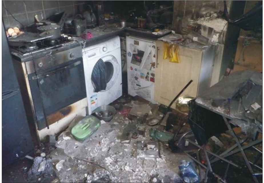
The damage caused to one flat after a scooter caught fire while being charged in a bedroom
